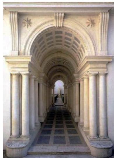
Figure 10: Arcaded courtyard of “Palazzo Spada”, Rome, F. Borromini 1635 [18]
